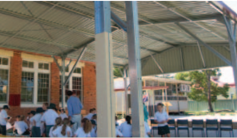
The new covered outdoor learning area at Wallabadah School.
