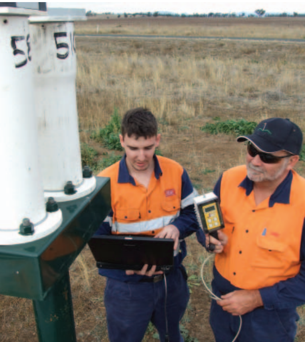
Gerard Gleeson and Sean Nolan from Australian Coal Industry Research Laboratory (ALS-ACIRL) download data gathered from a solar powered vibrating wire piezometer water monitoring bore. The data records continuous changes in water pressures at different strata levels.
