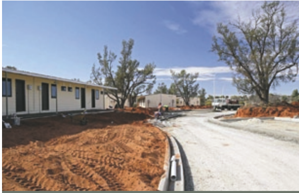
Plate 21.5 Construction of new contractor accommodation at Olympic Village
