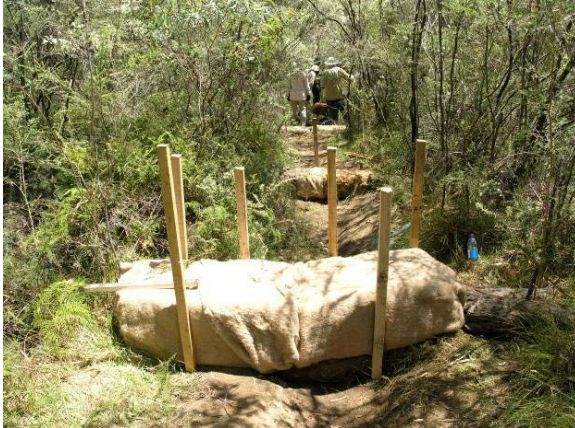
Plate 6-2 - Small Coir Log Dams Constructed at Intervals along an Incised Swamp with Jute Wrapping
