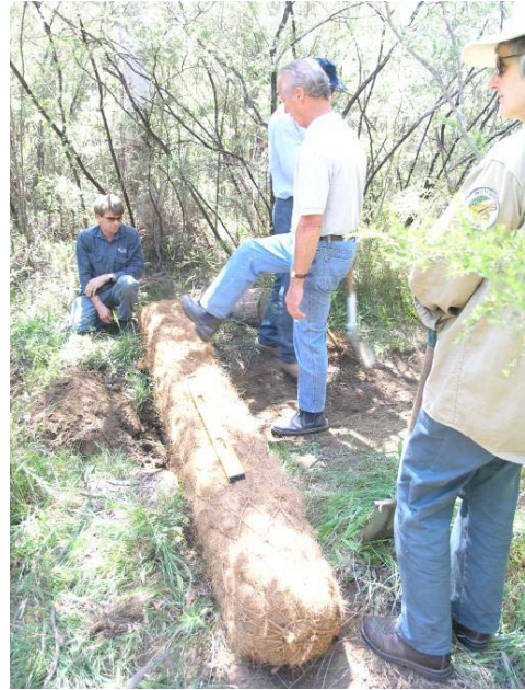
Plate 6-3 - Round Coir Logs Installed to Spread Water
