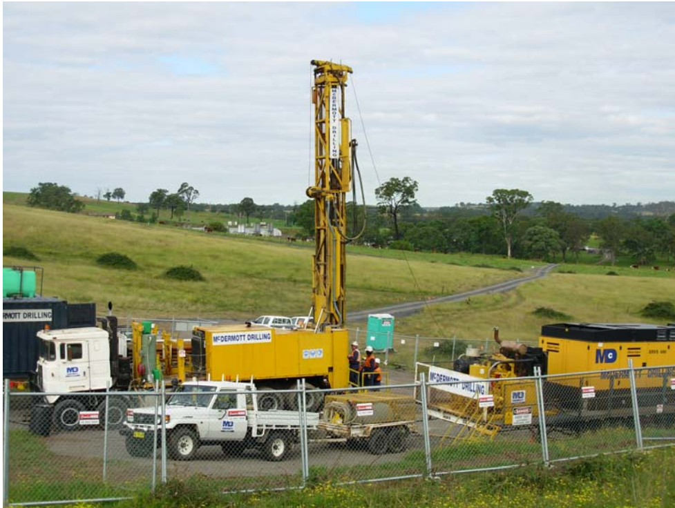
Photo 1. Borehole Drilling Plant at Appin, NSW
