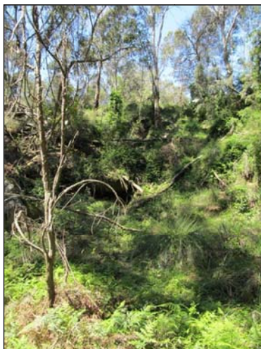
Plate 5: The dam wall constructed in the base of Leafs Gully taken from the downstream side and looking upstream.
