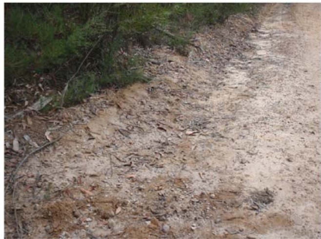
Figure 7.1 Results of rehabilitation of soil cracking in Fire Road 6C
