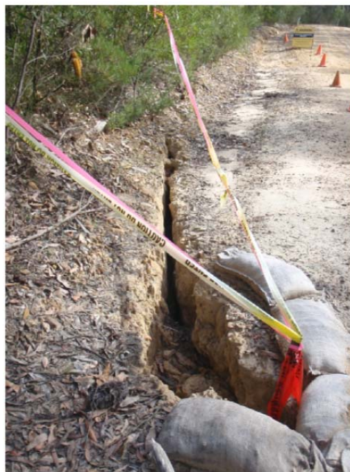
Figure 7.1 Results of rehabilitation of soil cracking in Fire Road 6C
