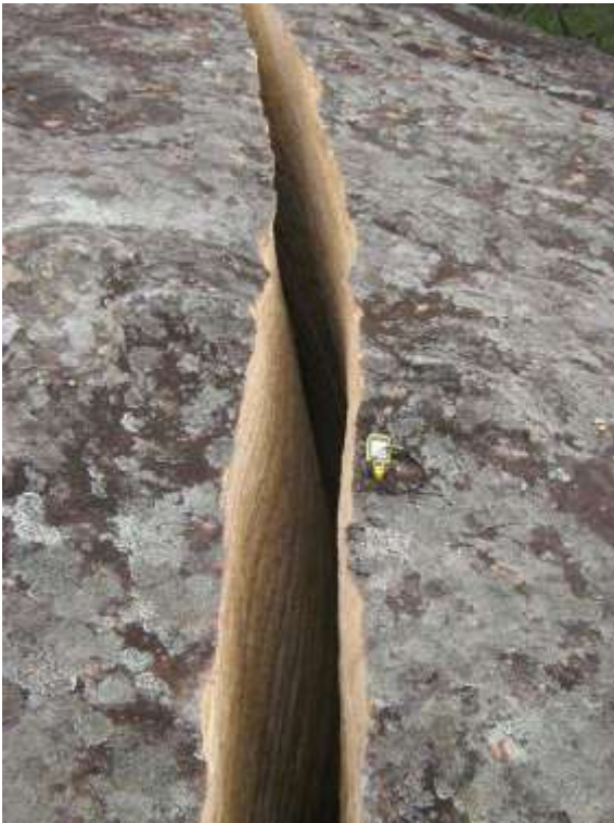
Plate 5: Cracks in surface bedrock observed within the Study Area.
