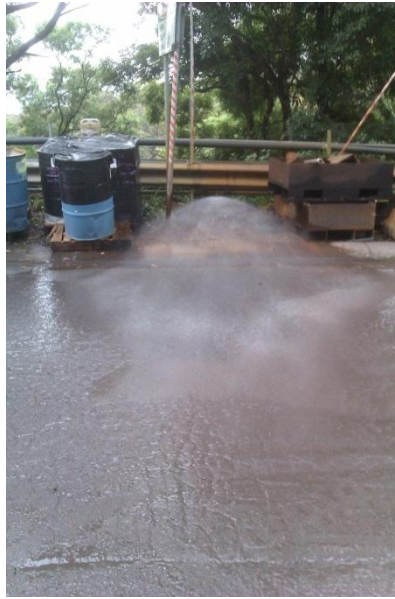
Figure 3.2: Image of portal road water sprays in use
