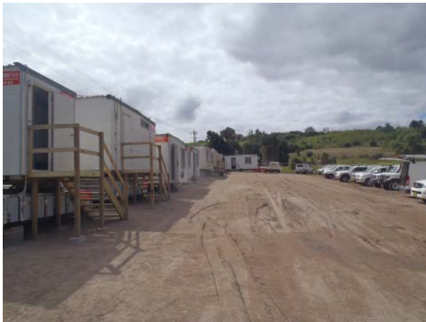
Figure 1. The access road Site Compound used to park light vehicles and provide temporary office facilities.
